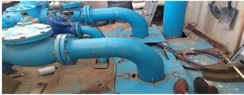
"Tanque cisterna rosa"
